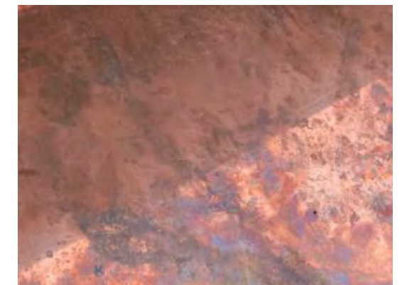
Copper Roof & Gutters
