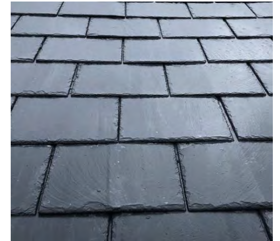
Slate Roof to match existing
