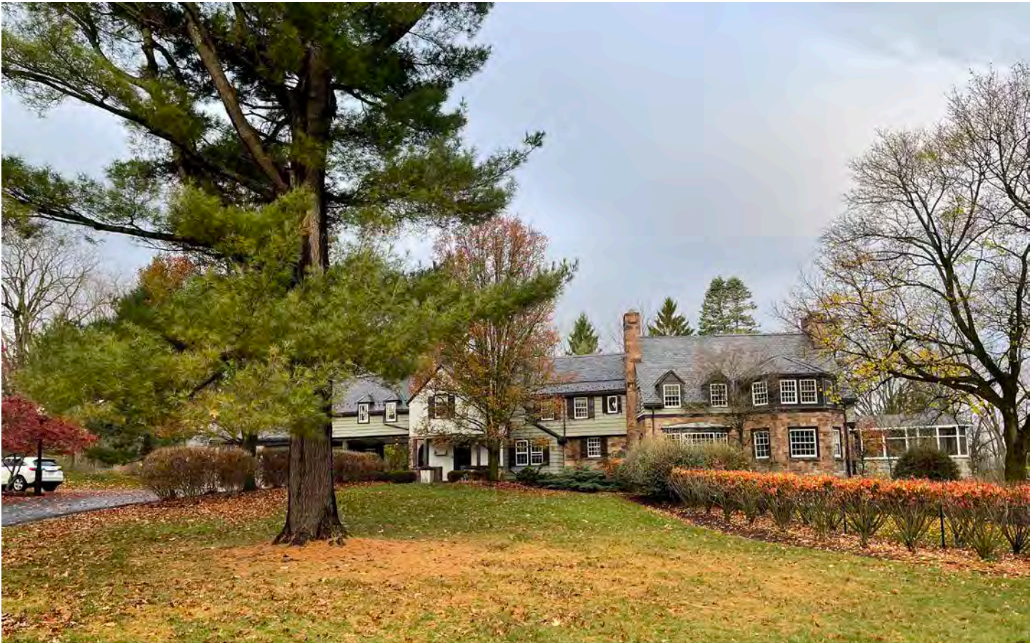
View existing screen structure and location of proposed screen room from side yard
