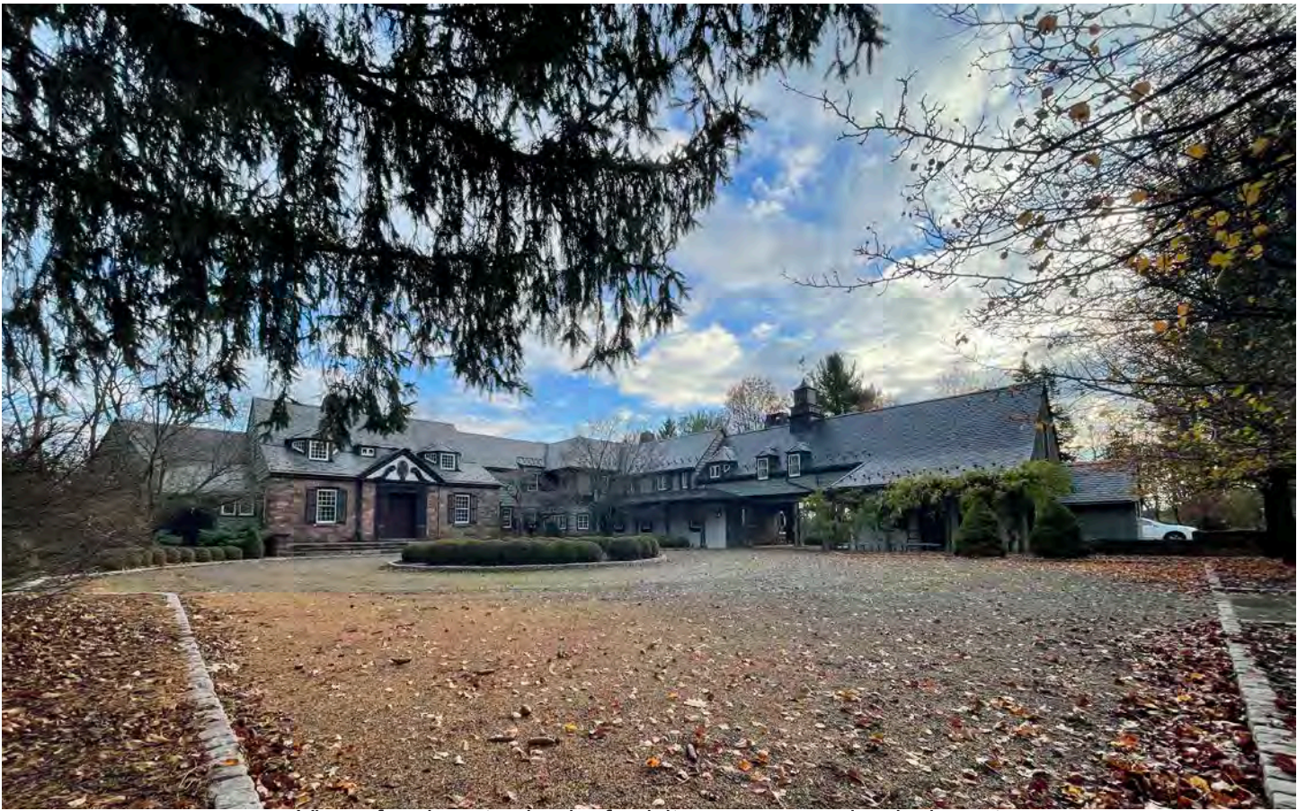
View of main entry, back of existing garage, and arrival court
