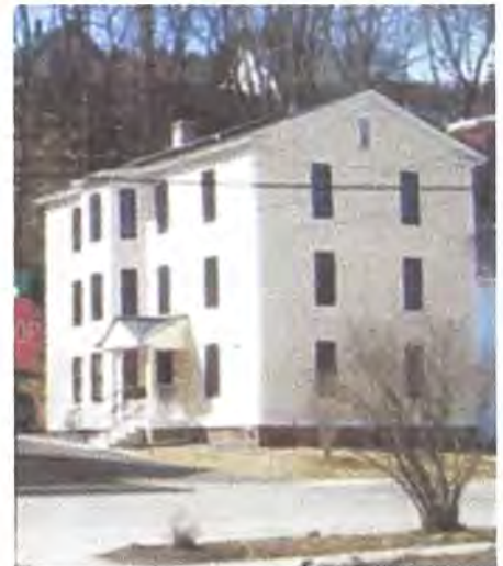
Low-profile solar collectors located on the south side of the gable roof are minimally visible.
