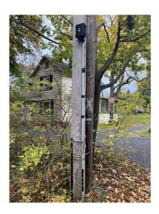
The State informs us that the cameras are a better alternative to tube setups because they are safer to install, safer for the traveling public, offer improved data accuracy, interfere less with snow and ice operations, and are less expensive.
