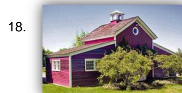
1 Mendon Center Road Gable roof - Reproduction Lusk Family Built 1999
