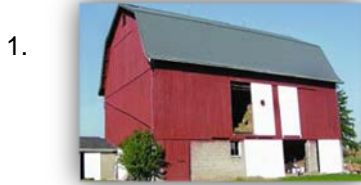
167 Willard Road Gambrel roof w/ basement James Willard Built mid 1800's
