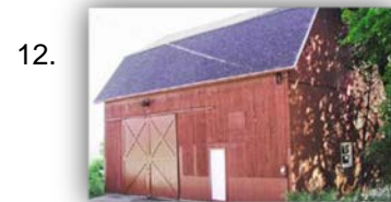
597 Mendon Center Rd Small English barn Hines-Stookey Built mid 1800's
