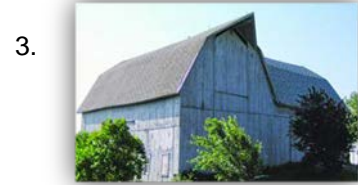
156 Mendon Center Gambrel roof Milton Tobey Built 1900
