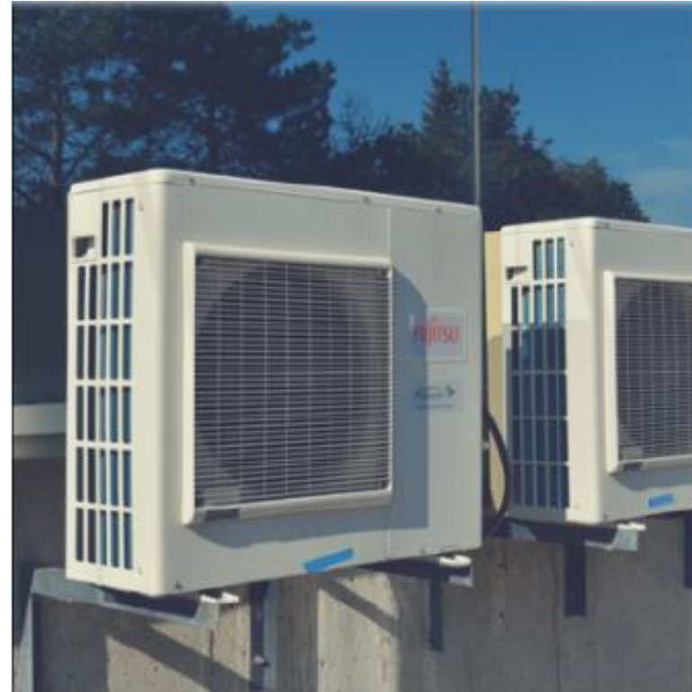
Refrigerant Management Program
